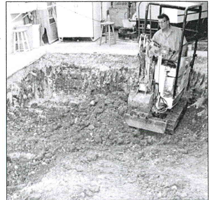
Enviroforensics worker removes contaminated soil from inside Bloomington Cleaners which was taken to a landfill near Detroit.
